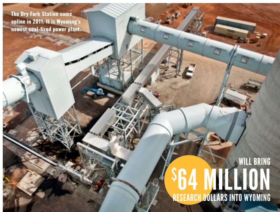
Researchers at the ITC use steel ducts to connect their equipment directly to flue gas emitted from the power plant.
